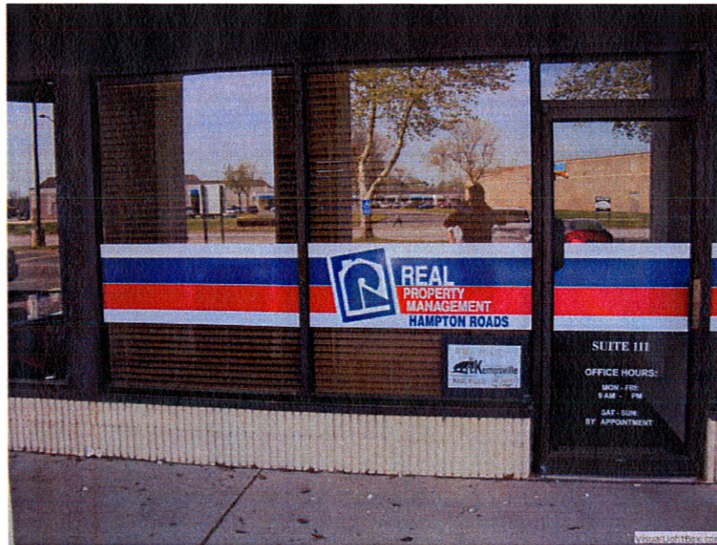
Figure 20 (4) Permanent Window Sign
